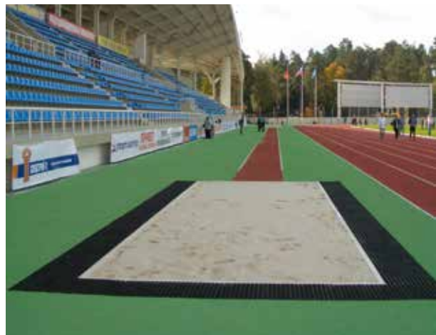
Sand pit with sand trap channels
